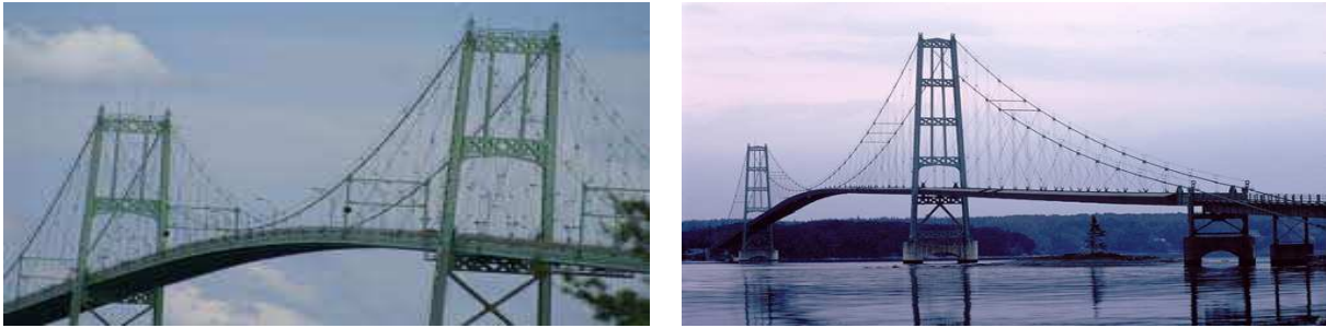
Figure 19: The Thousand Islands Bridge (left) and the Deer Isle Bridge (right).
