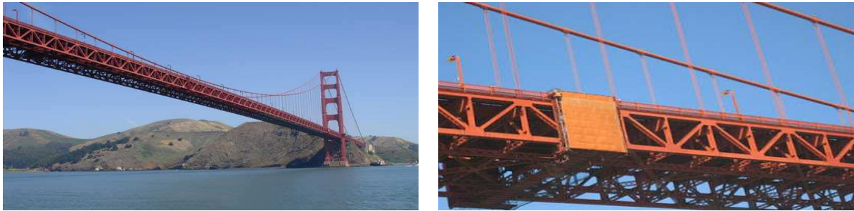
Figure 4: Girder at the Golden Gate Bridge.
