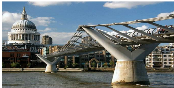
Figure 9: The London Millennium Bridge.
