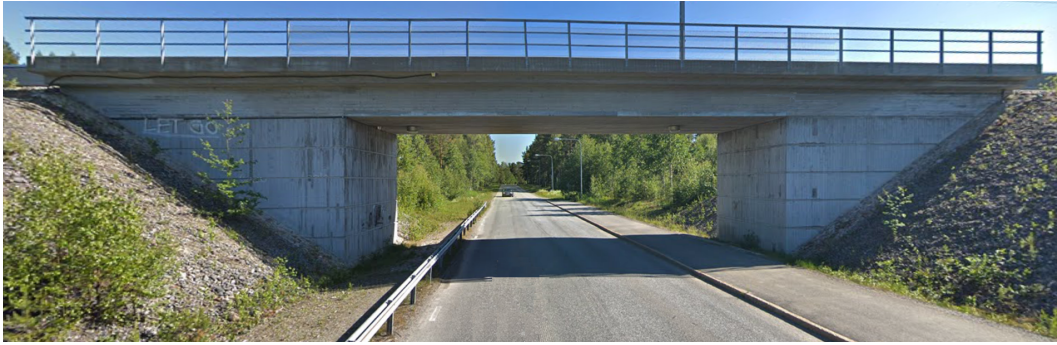
Figure 16: Hörnefors railway bridge.
