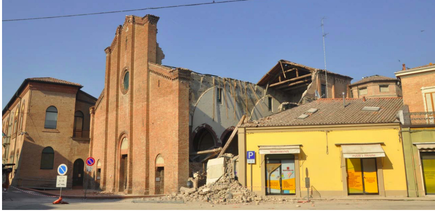
Figure 7: Collapse of the San Francesco Church (XV century), Mirandola. Courtesy of A. Penna.
