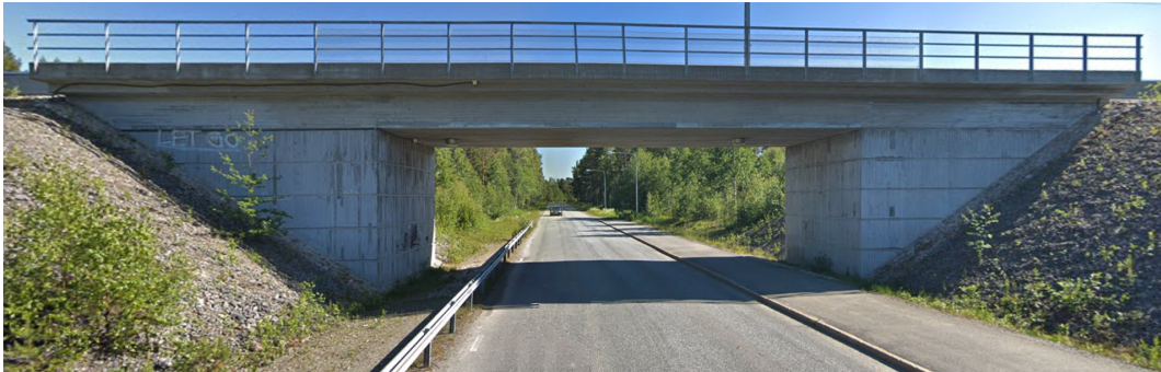
Figure 12: Hörnefors railway bridge.
