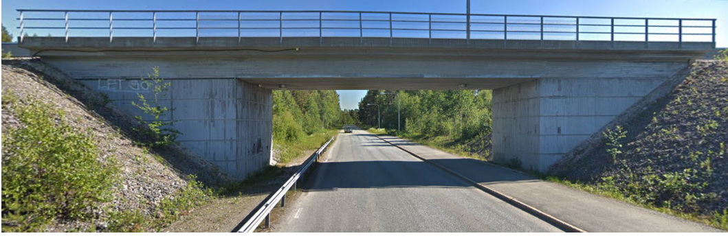
Figure 9: Hörnefors railway bridge.
