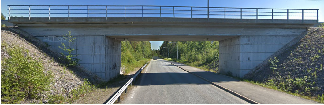
Figure 10: Hörnefors railway bridge.
